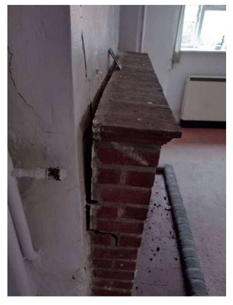
3. The ornate brick arched fireplace mantle has shifted and the brickwork is now loose and easily removed and represents a risk of complete detachment and falling to floor level. It should be repaired.
