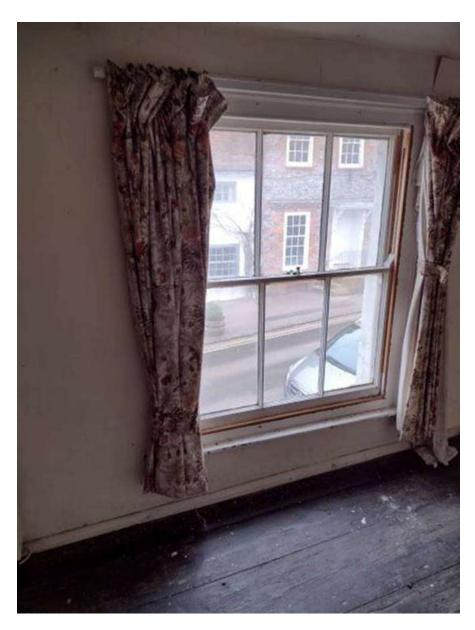
5. Low level glazing in the bedroom should be checked for compliance with Part K of the Building Regulations in relation to safety glass in high risk locations. Consideration should also be given as to any guarding required to prevent children from falling.
