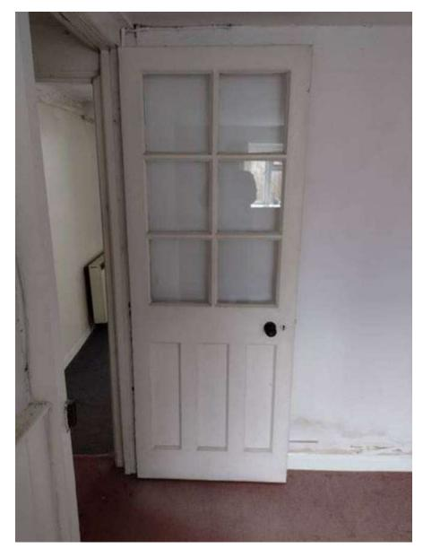
4. Glazing to internal doors should be checked for compliance with Part K of the Building Regulations in relation to safety glass in high risk locations (such as doors).
